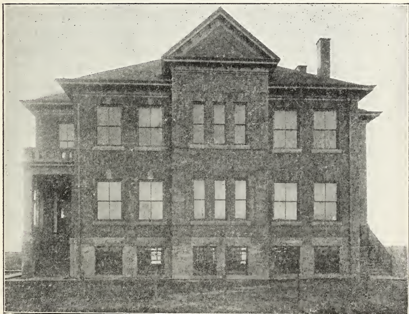
TRADES BUILDING, WESTERN UNIVERSITY.
